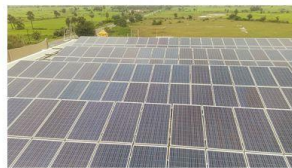
150KWP IN ODISHA, RCC ROOF TOP INSTALLATION
